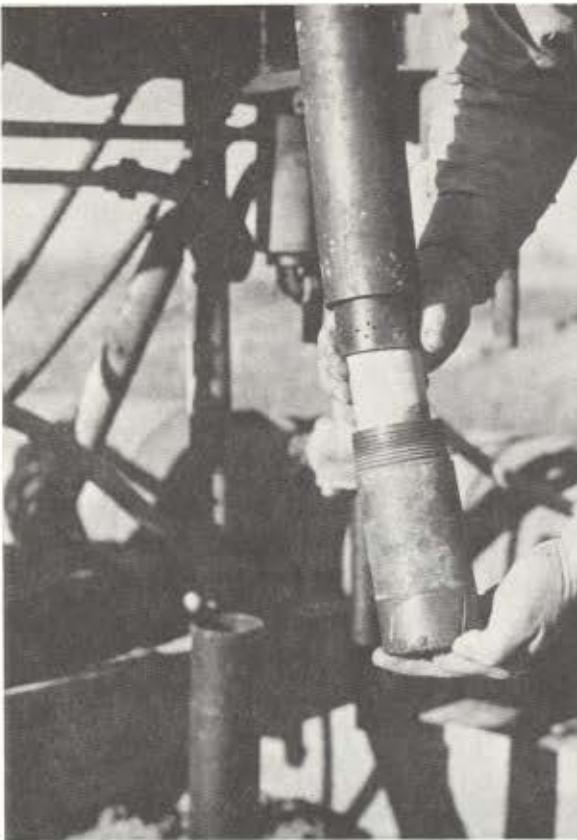
A CORE-DRILL BIT is pictured with a core of clay that was recovered after the bit was unscrewed. A core of this type yields a truly representative sample of the clay being prospected. Circa 1940-45.
