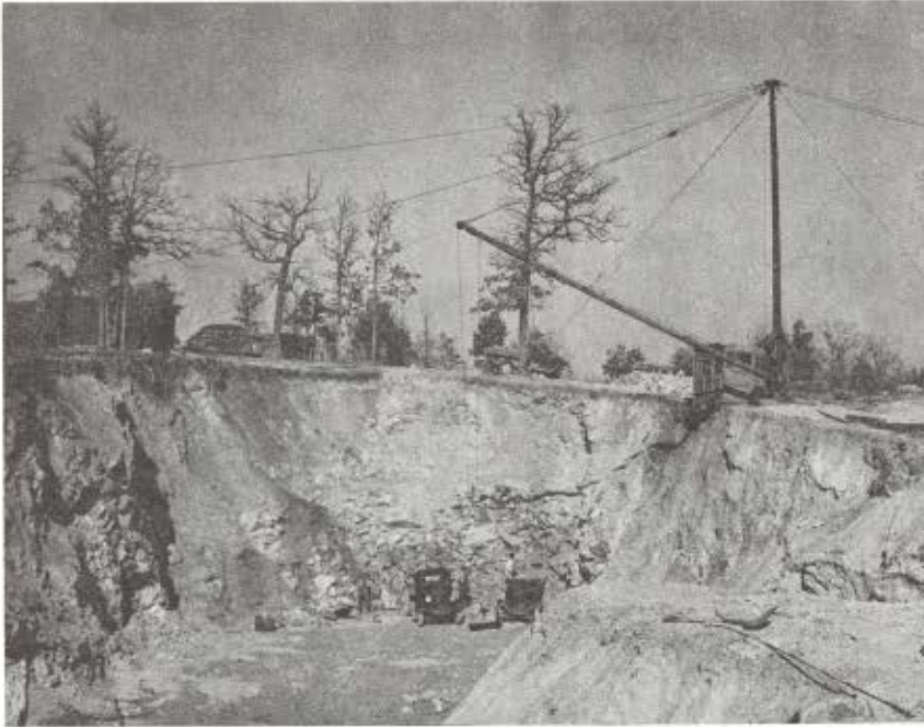
A "STIFF-LEG" HOIST was used to lift clay to a stockpile and onto trucks at the rim of this pit near Belle, Mo. The power to lift the clay was generated by a motor salvaged from an automobile. Photo, about 1930.
