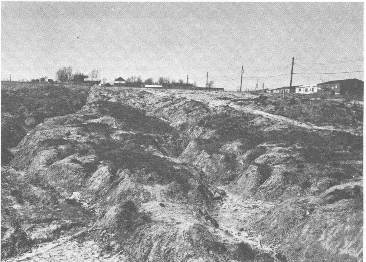
Figure 12. Erosion of planned development site after vegetative cover has been stripped.
