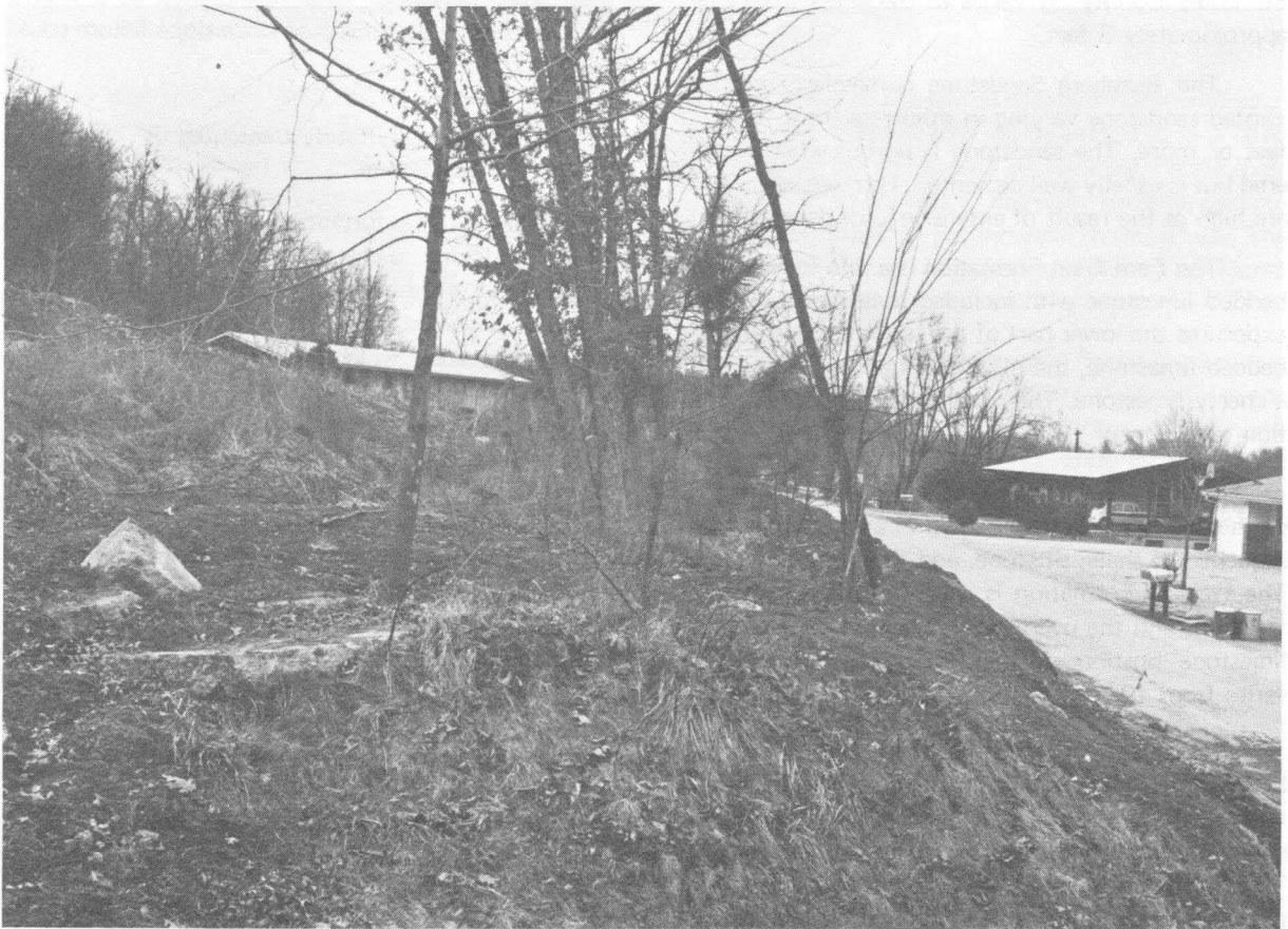
Figure 8. Leaning trees indicating soil creep over shales.
