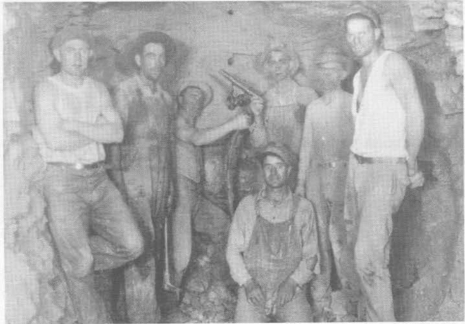
Figure 9. Tunnel excavation crew poses for a photograph during drilling operations for the Missouri Valley Tunnel, circa 1925.
