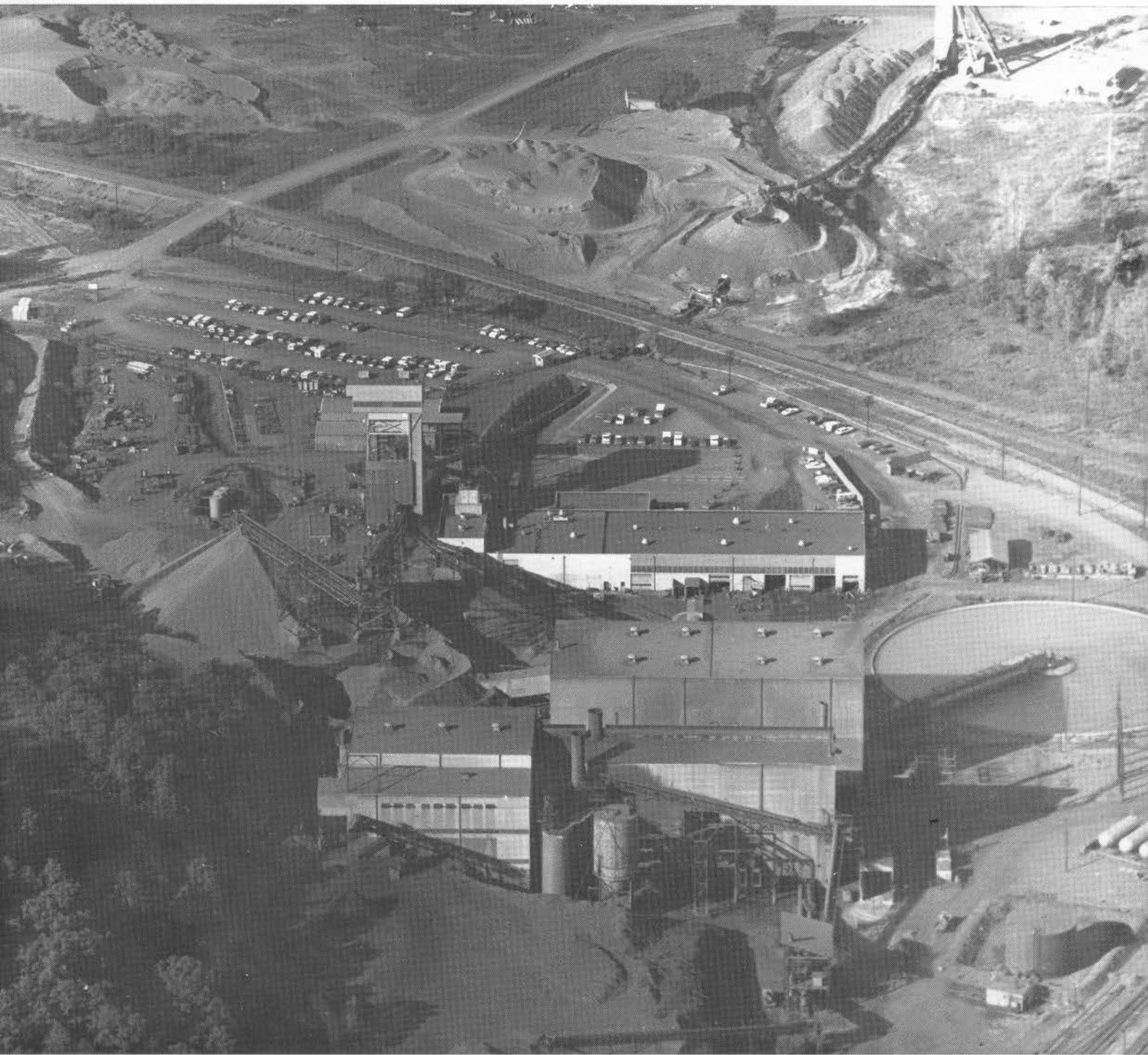
Figure 33. *Panoramic view southwest of the Pilot Knob Pellet Company's mine and pelletizing plant (SE $\frac{1}{4}$  NE $\frac{1}{4}$  and N $\frac{1}{2}$  SE $\frac{1}{4}$  sec. 30, T. 34 N., R. 4 E.). Production shaft is near the left center of the picture; building in foreground is the pelletizing plant. This mine-mill complex is 1800 ft east of mileage point 52.6. Photo by Jerry Vineyard.*
