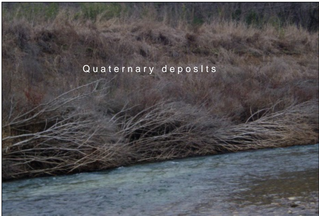
Figure 25. Park Service placed tree revetments to mitigate erosion of unconsolidated Quaternary bank deposits. From Smart and Doerr (no date).
