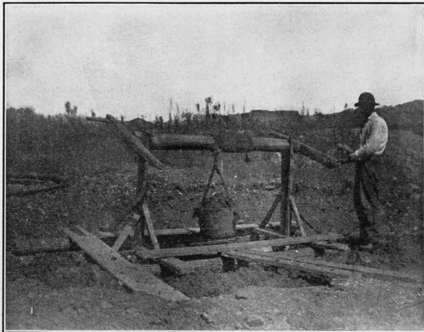
HAND WINDLASS HOIST IN OPERATION.
