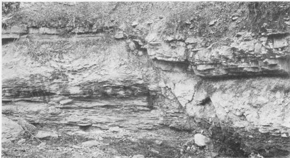
Fig. 1. Faulting in Hertha limestone.
