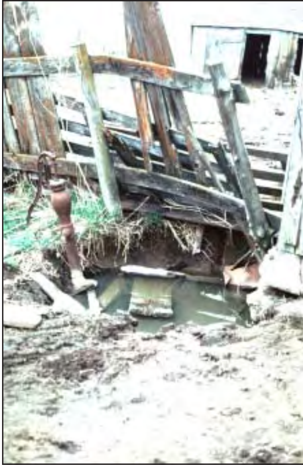
Abandoned and forgotten hand-dug well in farm lot. Notice rotted cover and old hand pump. Photo by Jim Vandike.
