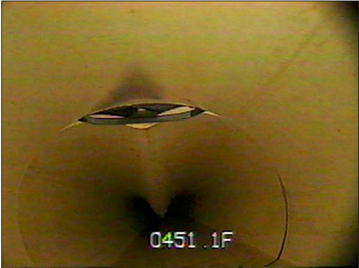
Pipe damage as seen by the inspection camera. Source: Dam and Reservoir Safety Program.
