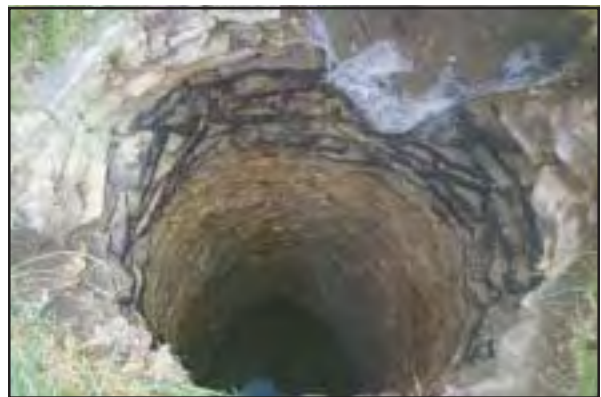
Looking into an old hand-dug well with cover removed. The well is approximately 4 to 5 feet in diameter and 30 feet deep. It is lined with fieldstone. Photo by Bruce Netzler.
