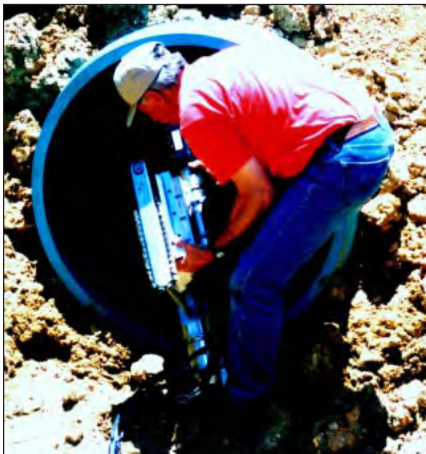
Pipe inspection camera being placed into spillway pipe. Source: Dam and Reservoir Safety Program.
