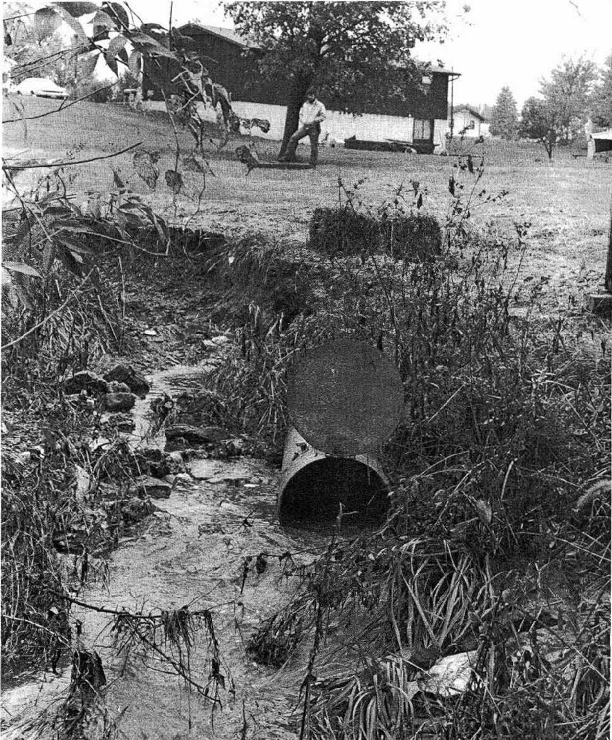
Figure 10 -- Herberlie Resurgence discharges through an inclined tube linked to a vertical rise pipe (upper center).
