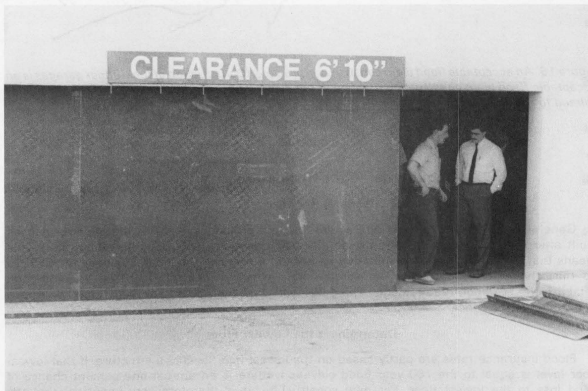
Figure 15. Steel flood door partly closed at garage entrance. (photo by Nick Decker)
