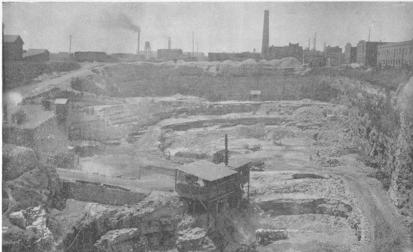
STIEFEL AND RUCKERTS QUARRY—LOOKING SOUTH. Illustrating a large and deep sunken quarry in distinction to a bluff quarry.
